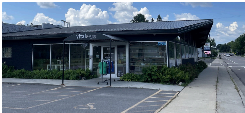
Street-facing storefront on N. Stevens Street, with on-site parking.
